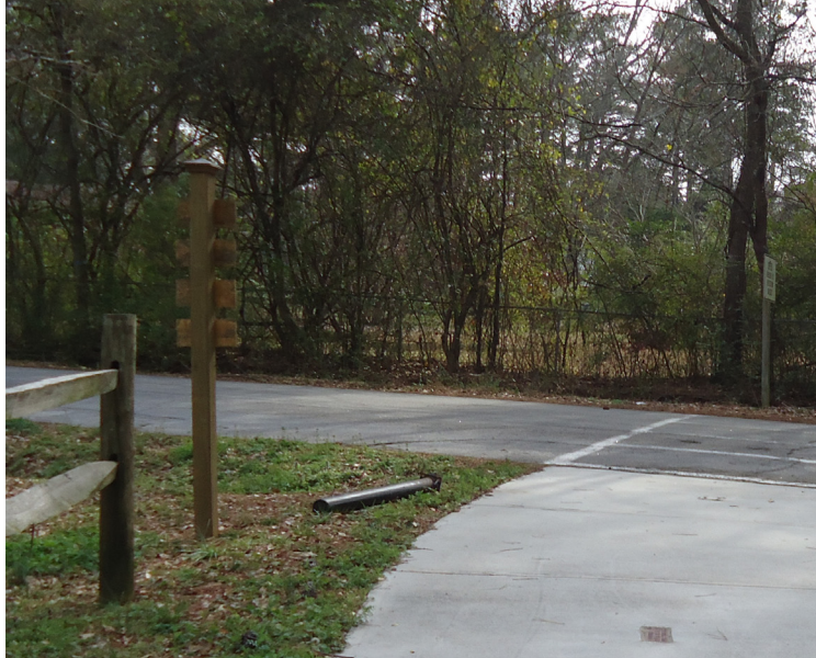
Misplaced bollards are a sign that the trail requires more upkeep. There are also crosswalks that need to be repainted to improve driver visibility.
